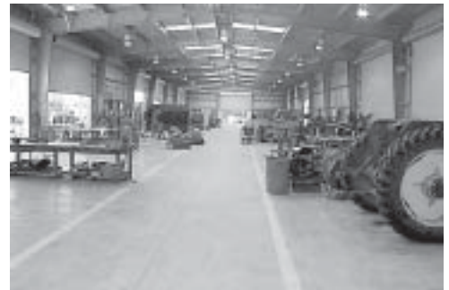
Big projects are no problem in our 15,000 square foot assembly building.
